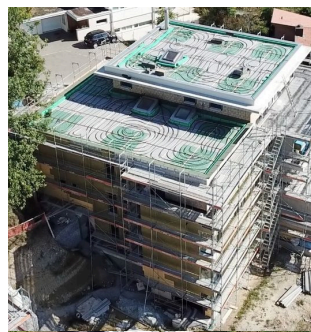
Laying the external collector circuits on a flat roof
